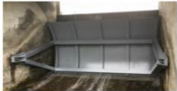
Tainter Gate installed at Lower Malad Lake, Utah 4,000 Lbs
